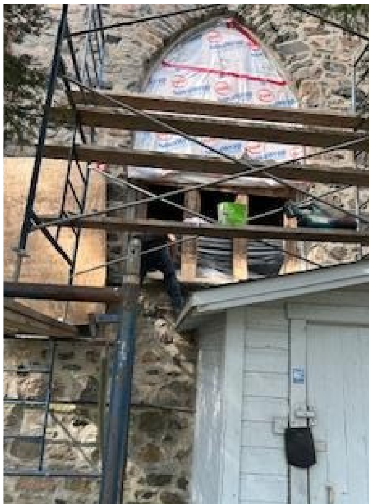
Construction Benoît Moreau Inc. restored the main window. Photo: Johanne Jutras.
